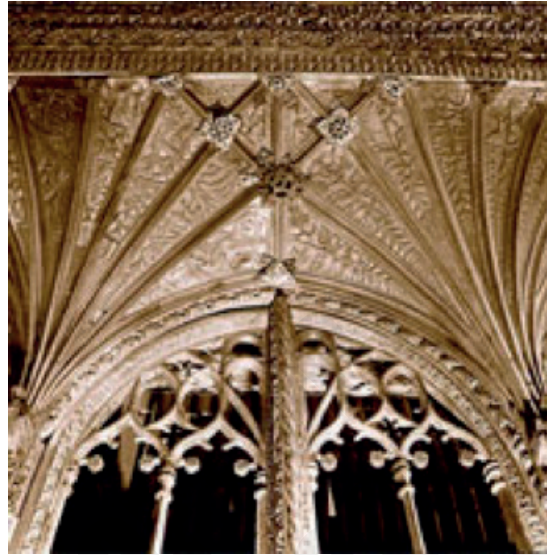
Detail of the Gothic rood screen, c.1500
